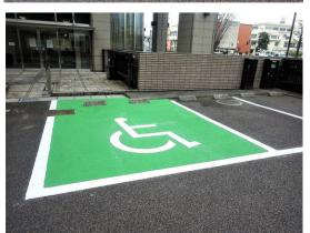
In parking spaces for people with disabilities, we improved visibility by implementing color paving, which is made by pulverizing and adjusting the particle size of waste tiles that used to be reclaimed as aggregate, and adding pigments to a special emulsion.
